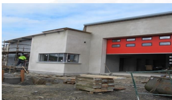
New Graiguenamanagh Fire Station Works to be completed 2018
