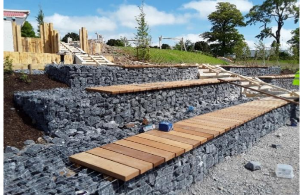
The terraced seating area in Ferrybank Neighbourhood Park. As the site is on elevated ground, there are great views of Ferrybank and Waterford City from this area.
