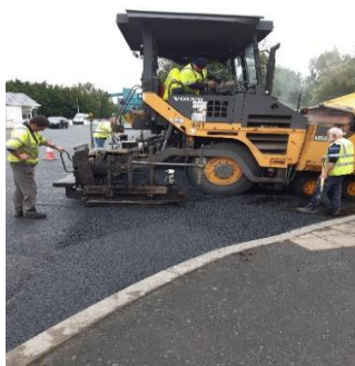
Paving works at Kilkenny Road Callan
