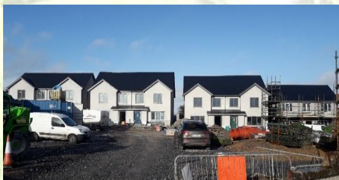
Breaghagh Place, Piltown – 17 units under construction
