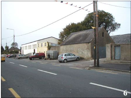
Photo 6: East side of Main Street - opportunities for redevelopment and the creation of more active uses along the street front.
