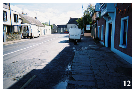
Photo 12: Quality of footpath in centre of village is in poor condition.
