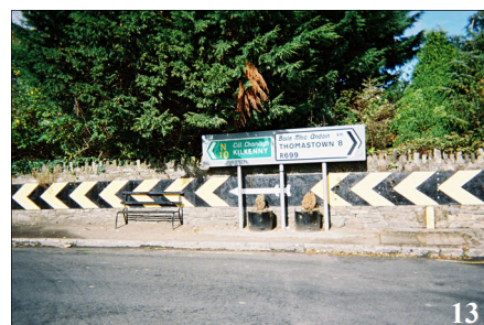
Photo 13: Street furniture—planters and seat—are in relatively poor condition.
