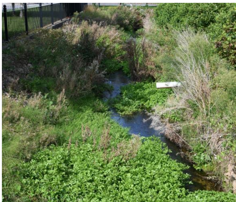
Plate 5. Section D showing discharge pipe from bank.
