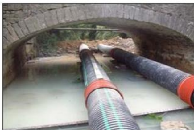
Figure 6.17 Flow Piped from upstream to downstream (Source: IFI Guidelines on Protection of Fisheries during construction works in and adjacent to waters 2016)
