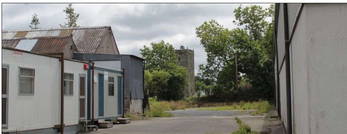
Plate 9-5: Stream is culverted under Arrigle business park
