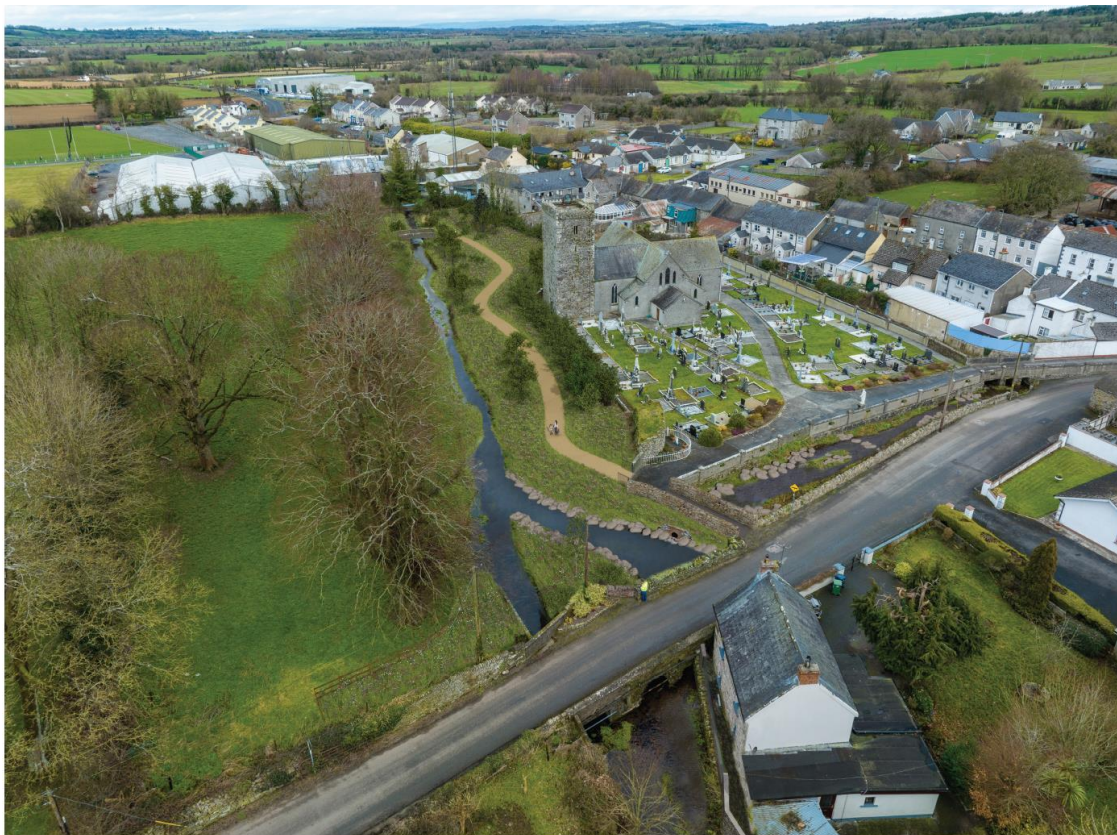
Figure 9-11 – Aerial view of proposed works around Ballyhale Church prepared by Chris Shackleton
