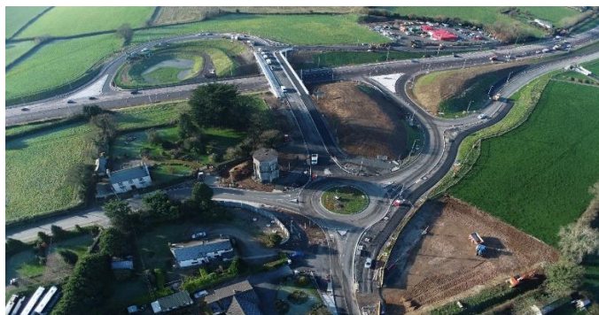
Overhead drone footage of the compacted grade separated junction.
