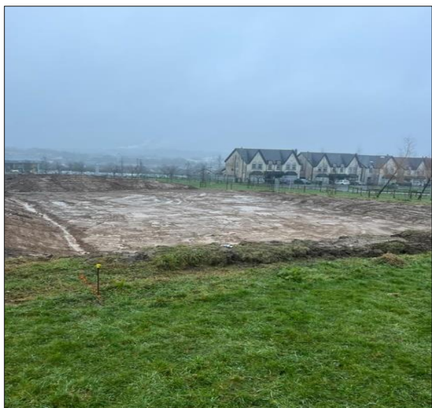
Excavation works for new MUGA, Ferrybank Park
