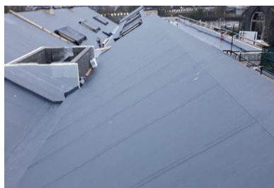
Installing frames of Roof lights commenced.
