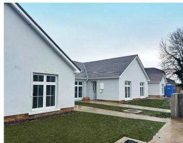
5 UNITS, BERKELEY DRIVE, FERRYBANK
