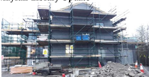
Fixing of insulation and flashings to flat roof ongoing.
